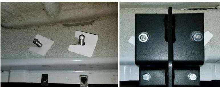
Using the 3" U-Bolt put it through the top 2 mounting holes and secure with (2) plastic bolt retainer.
