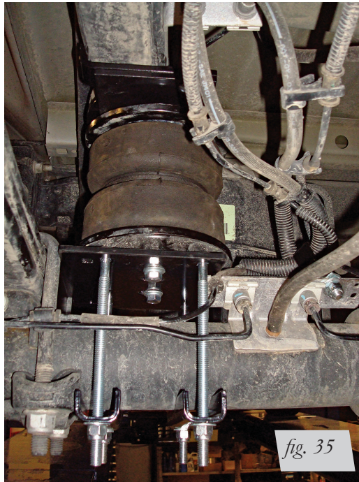
Left side (driver): rear view of installation.
